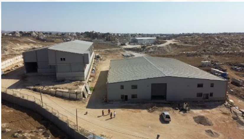
Figure 4: Plastic Factory Current Status (right) with the Artisanal Dairy Factory (left)
